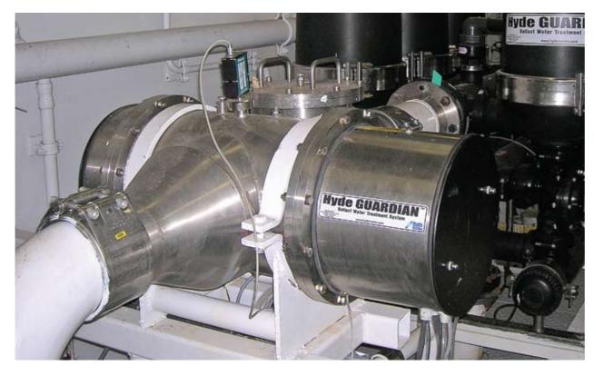
The Hyde GUARDIAN uses a high intensity ultraviolet (UV) treatment as a means of disinfection. The UV chamber is carefully designed for minimum pressure drop, maximum retention time, and compatibility with the marine operating environment.
