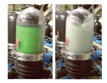
inlet and opens the drain. By removing the differential pressure in the system, the spine piston rises up releasing the compression on the disks. Tangential jets of clean water are pumped at high pressure in the opposite direction through nozzles at the center of the spine. The disks spin free and clear, loosening the trapped solids. Solids are quickly and efficiently flushed out through the drain and immediately overboard. As this water contains only organisms that were recently picked
